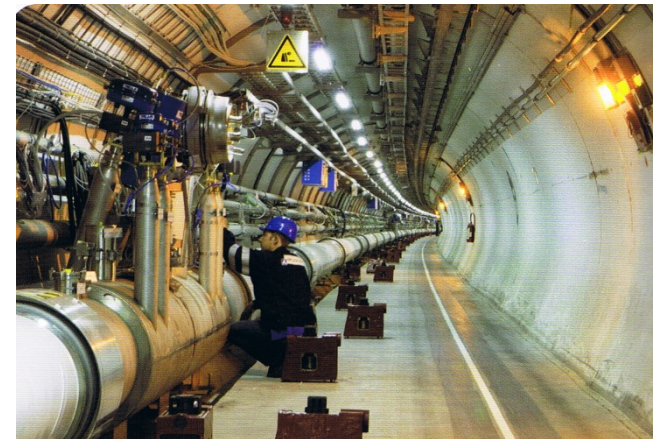
The 27 kms lines used to transfer 1.8K Helium LHC CERN
